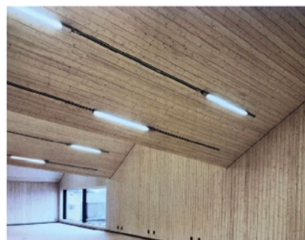
Fig.38: (left) Showroom with wooden roof, Visitor Center in Kosterhavet National Park, White arkitekter, Sweden, 2012
